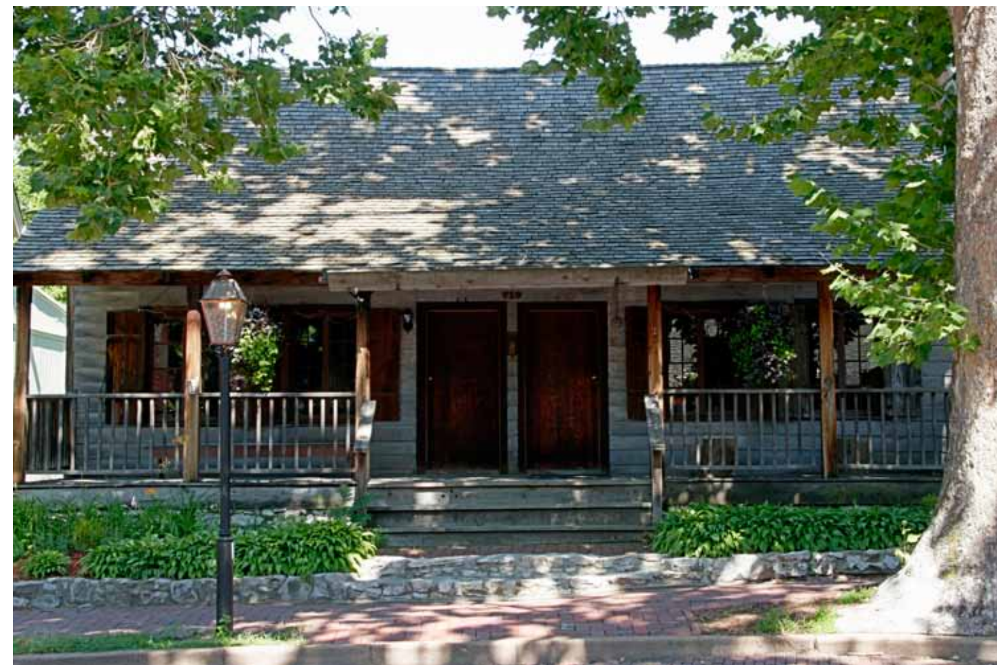
719 South Main - Original Construction circa 1769
