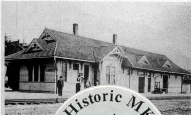
This is how the depot looked that year at the foot of
