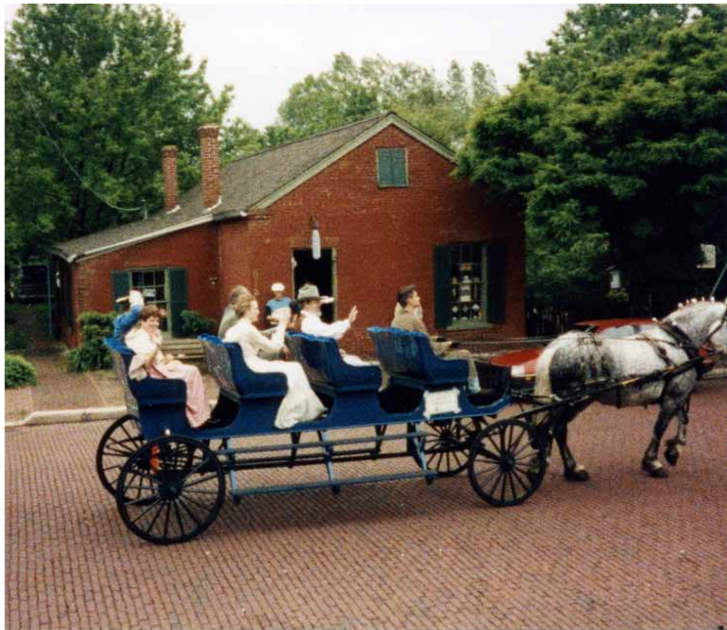
912 South Main - Original Construction circa 1850
