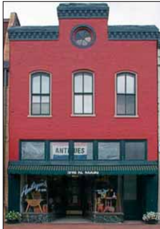
To restore the building at 319 N. Main, Pitman removed boards that had been placed over the round window at top and the small square windows just over the awning. At left are an old photo of the building and a photo of the restoration work.
