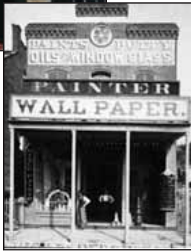
To restore the building at 319 N. Main, Pitman removed boards that had been placed over the round window at top and the small square windows just over the awning. At left are an old photo of the building and a photo of the restoration work.
